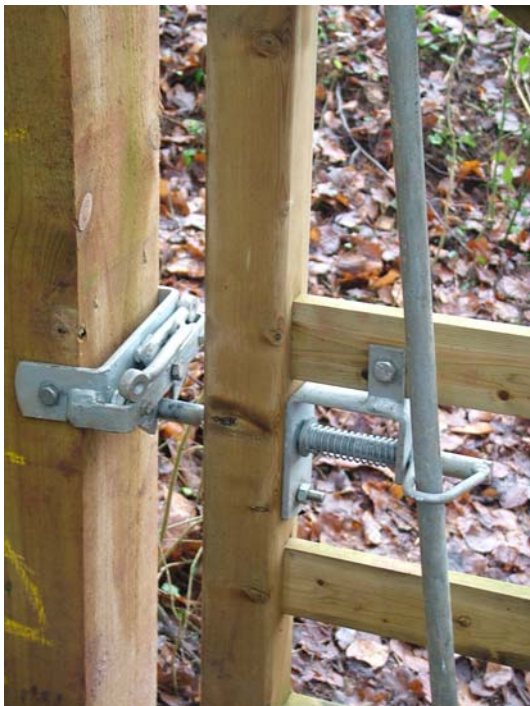
Two Way Latch Detail
