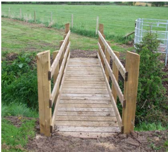
Open standard footbridge with level footpath approach
