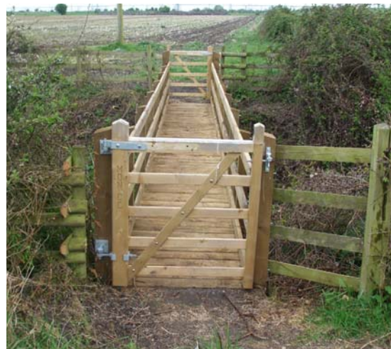
Gated standard footbridge to maintain stockproof paddocks
