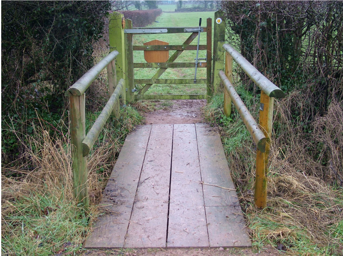
Timber Sleeper Bridge
