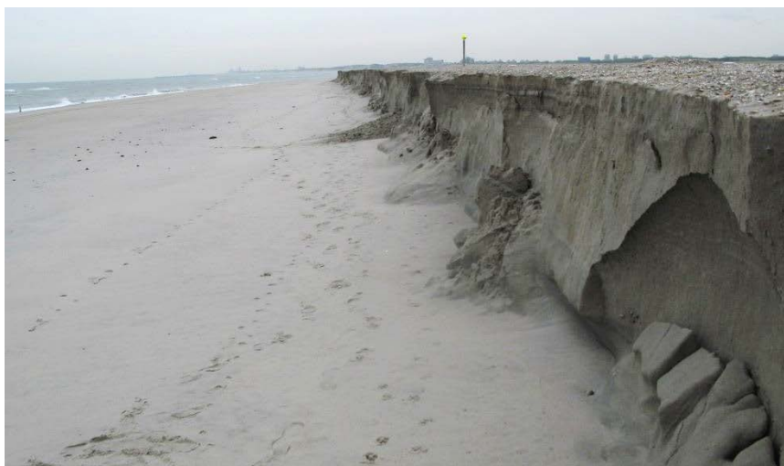
Fig. 7. Beach cliff on NW side of the Sand Motor mega nourishment (photo October 8, 2014).
