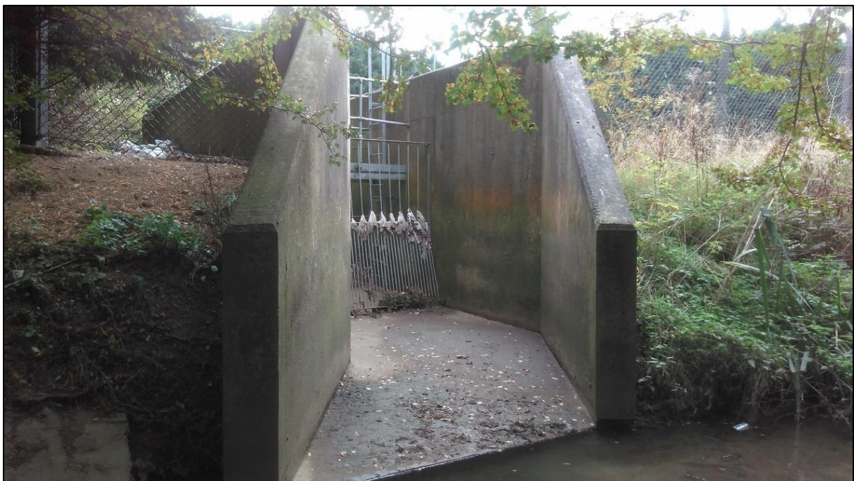
Figure 2. Photo 1 – Manthorpe Mill high level CSO outfall
