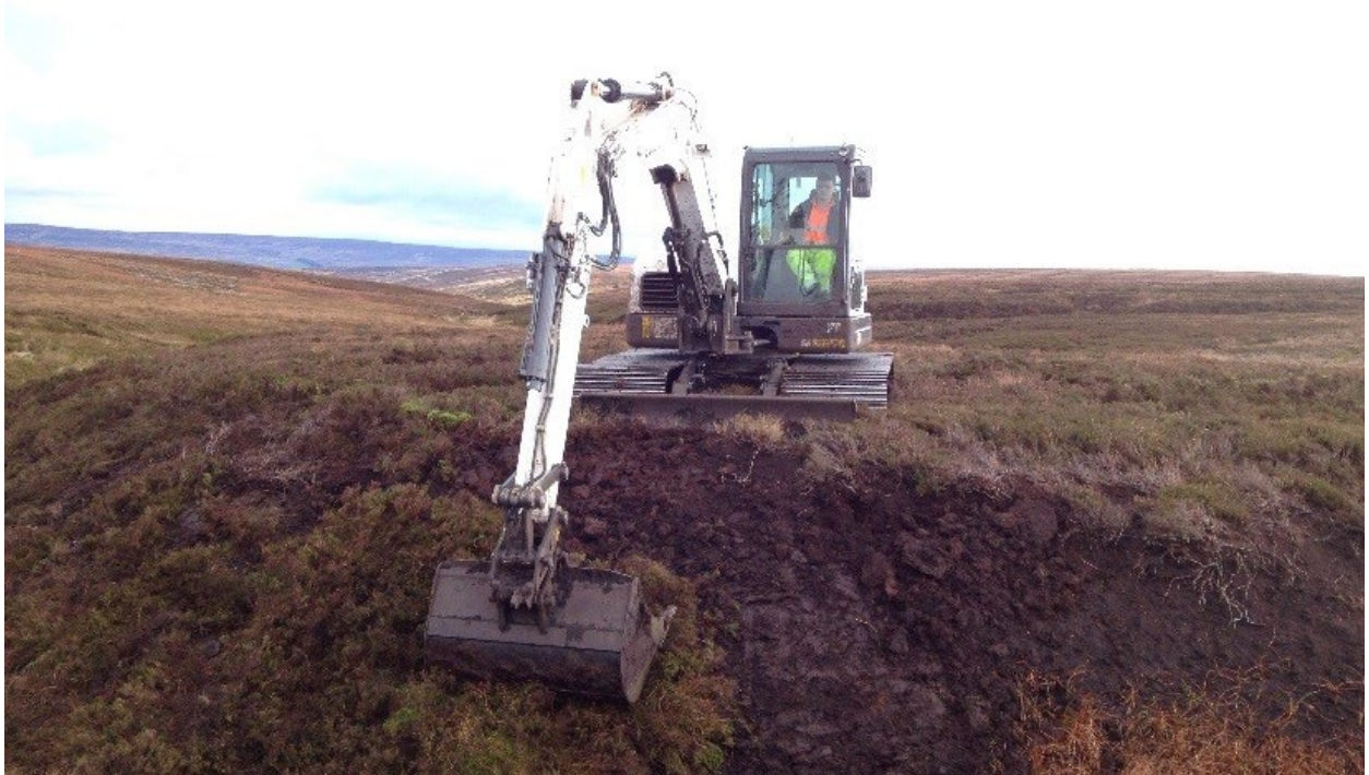
Reprofiling and turfing a peat hag, Ramsgill. © Rosie Snowden
