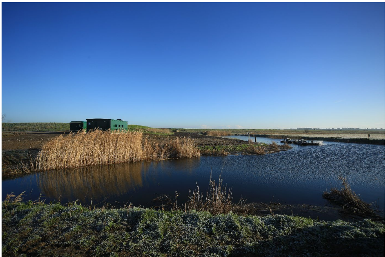
A pump house on the Felixstowe Hydrocycle
