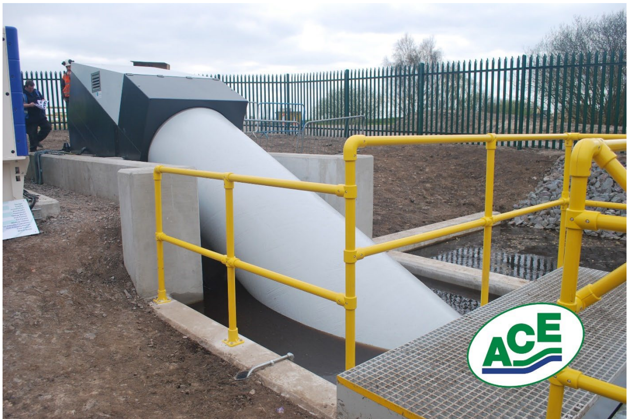
Archimedes screw pump at Thorne Moors
