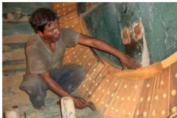
Figure 10. Installation of wooden sectors to improve drainage of floats
