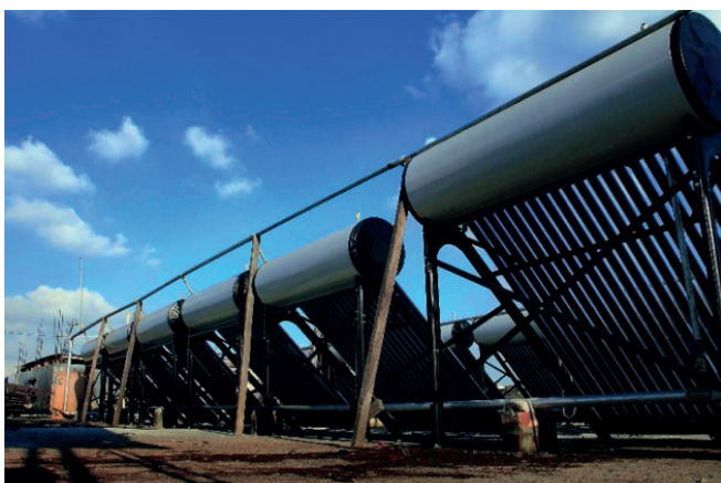
Figure 98. Solar collectors installed in a tannery under a UNIDO project in Bangladesh
