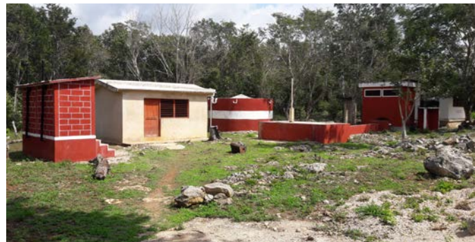
Figure 21. Ecotechnologies at a community school. From right to left: dry toilets, cisterns and a biodigester. ©Photograph by Gonzalo Merediz, Amigos de Sian Ka'an.
