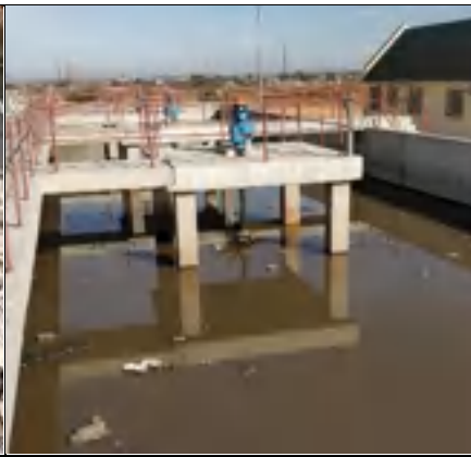
Three of 4 aerators are not functional, long lead times before equipment is repaired. No operational control
