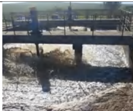
Aerators in new reactor functional, not in older module due to cable theft
