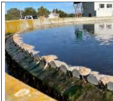
Good operational working of secondary settlers
