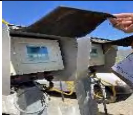
Flume with ultrasonic meter for inlet flow monitoring, verifying 44% of design capacity
