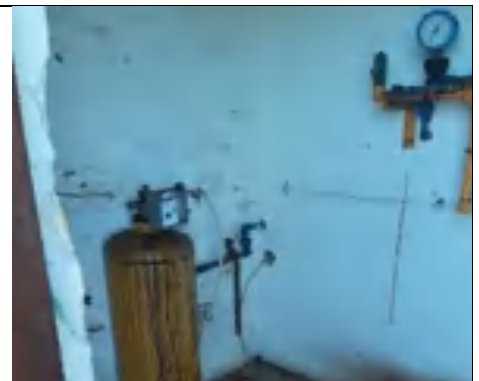
Chlorination room vandalised and stripped, not functional
