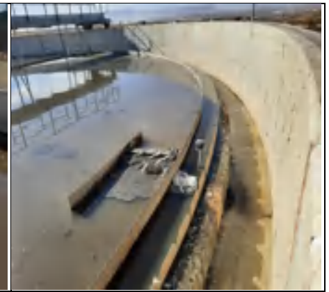
Scum withdrawal system not functional. Poor sludge settleability with pockets rising to surface
