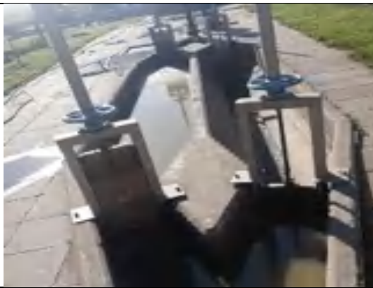
Flow meters and grit channels operational. Mechanical screen out for repairs, manual screen overloaded
