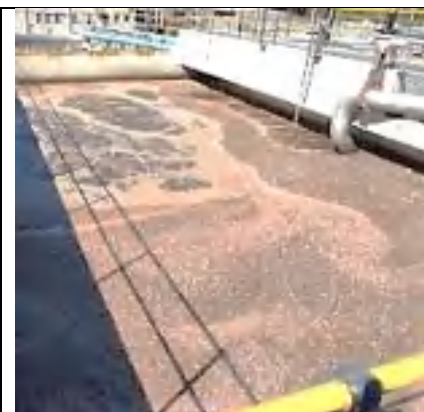
The plant uses fine bubble aeration in the bioreactors and in general a good distribution of air could be seen.
