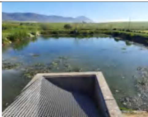
Dam receiving overflows is not in good condition. Sluice gates stolen and sludge build up noticed
