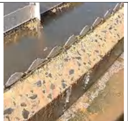
Minor corrosion on the concrete was seen in some areas and need to be addressed.
