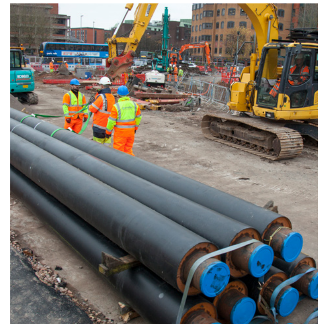
Redcliffe district heat network being built.
