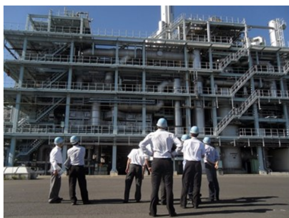
Figure 9 -Large-scale biochar production facility in Japan, processing 700 tonnes of dry sewage sludge into char.
