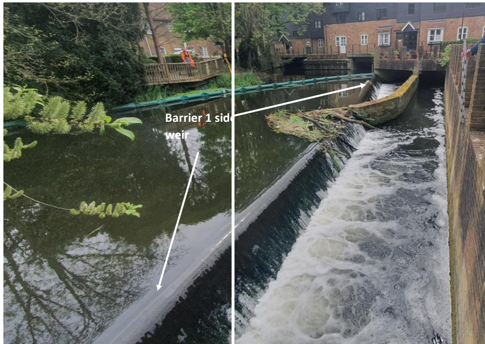
Figure 5. West Drayton Barrier 1 with barrier in place
