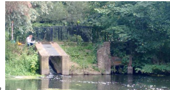
Figure 3. Barrier 1 to Fish Passage at West Drayton Mill
