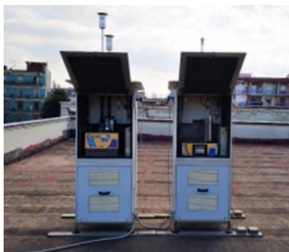
Environmental monitoring station installed in the Municipality of Pomigliano D'Arco
