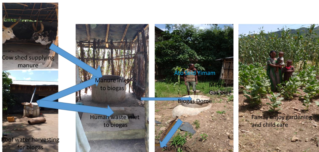
Photo 4. Showing the biogas plant and biogas inputs, outputs and process from manure supply to methane gas production at Mr Seid Yimam household. (Source: Zewdu Eshetu. 2020).
