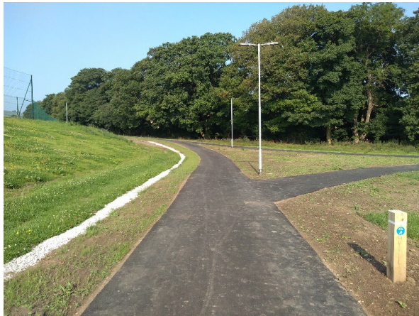
Figure 15.4 – Example of lighting on a shared route in Holywell
