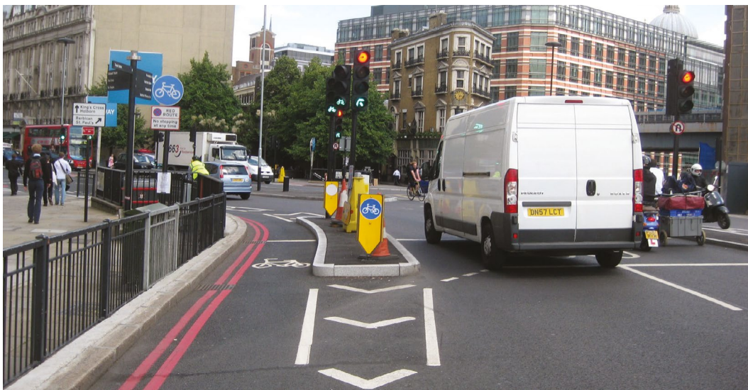
Figure 12.15 – Left slip bypass at signals
