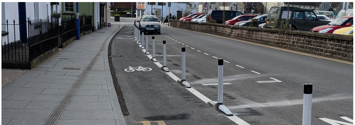
Figure 11.12 – Light separated cycle contraflow
