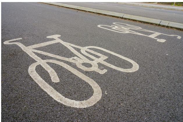
Figure 11.5 – Diagram 1057 painted onto carriageway
