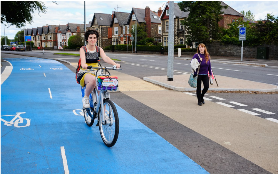
Figure 9.10 – Cycle track runs continuously through a side junction
