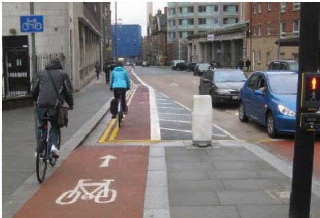
Figure 11.19 – Transition from cycle track to cycle lane, Liverpool
