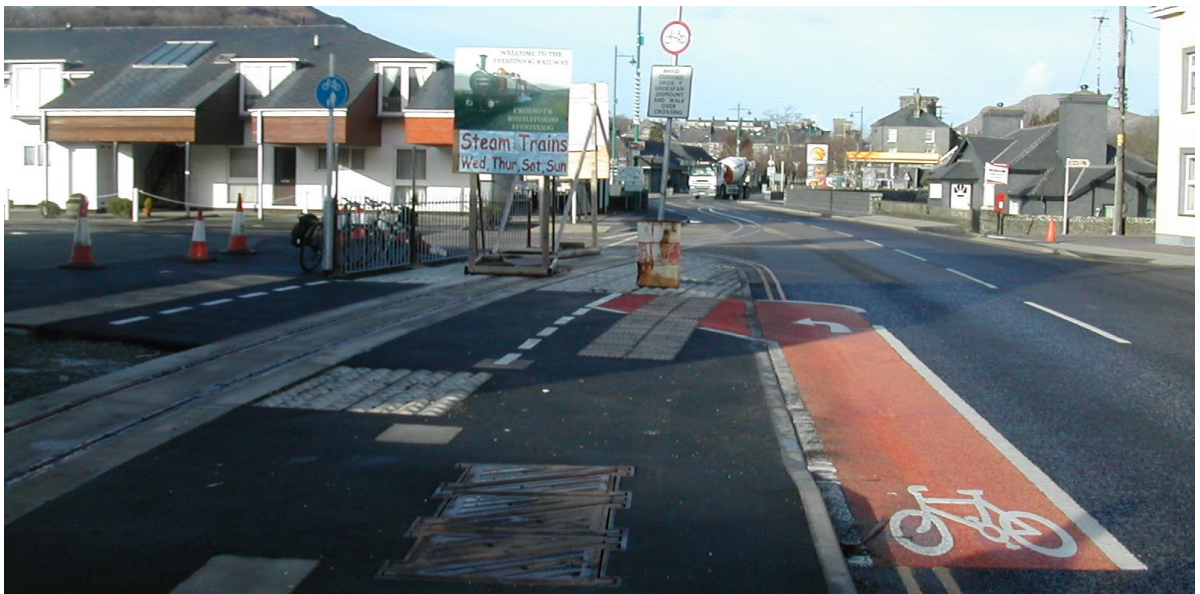
Figure 11.24 – Cycle route crossing heritage railway tracks which run along the carriageway
