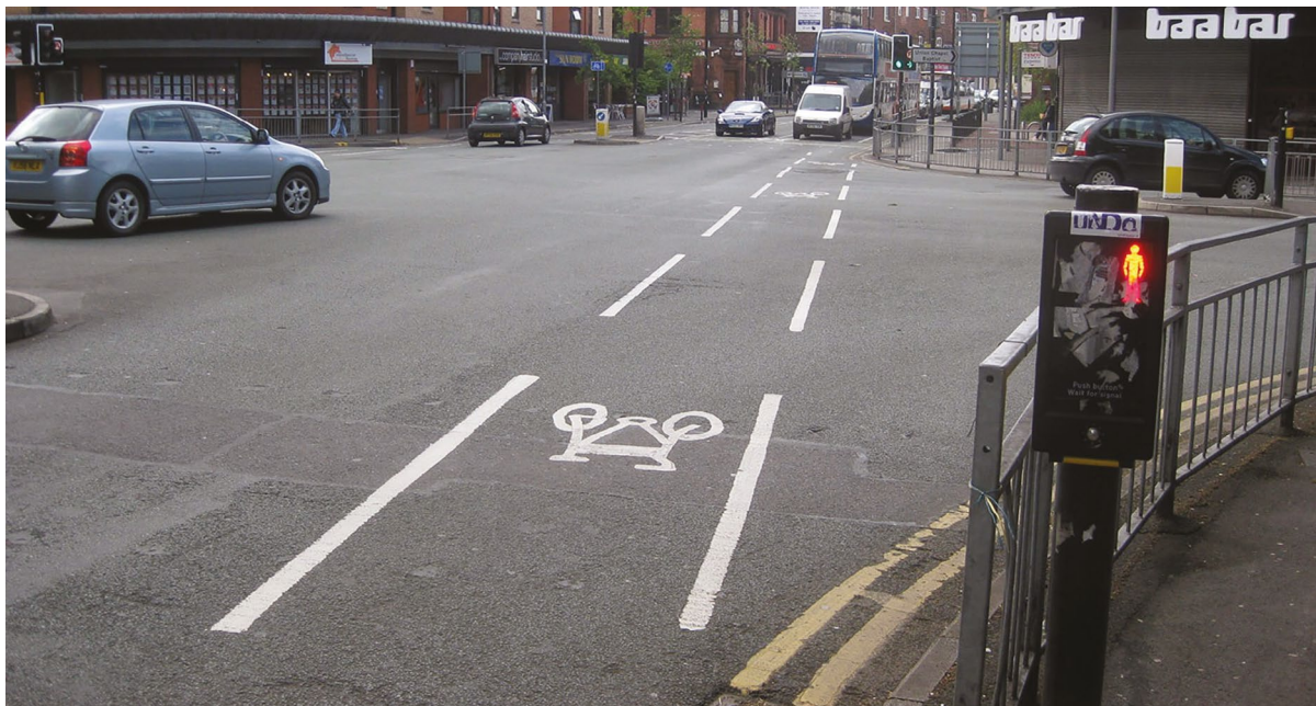
Figure 12.17 – Elephant footprint markings through junction
