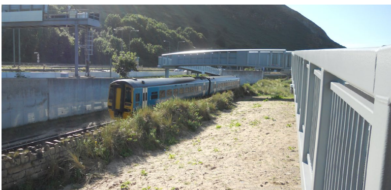
Figure 12.27 – Bridge with angled approaches, Conwy Morfa
