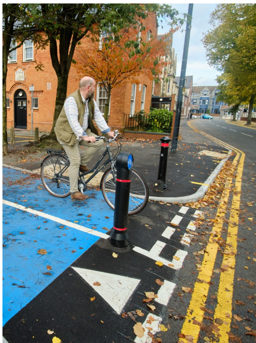
Image of modal filter, Riverside, Cardiff (note that a build out into the parking bay is also recommended to avoid vehicles parking across the dropped kerb)
