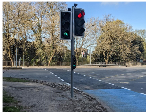
Figure 12.11 – Separate cycle stage with high and low level cycle signals
