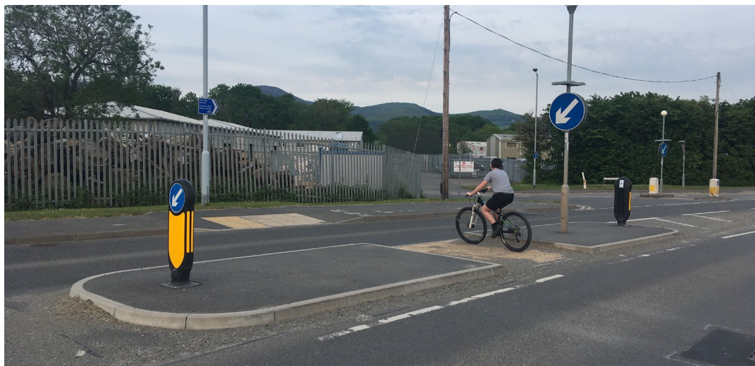
Figure 12.6 – Uncontrolled crossing with central refuge, Ruthin
