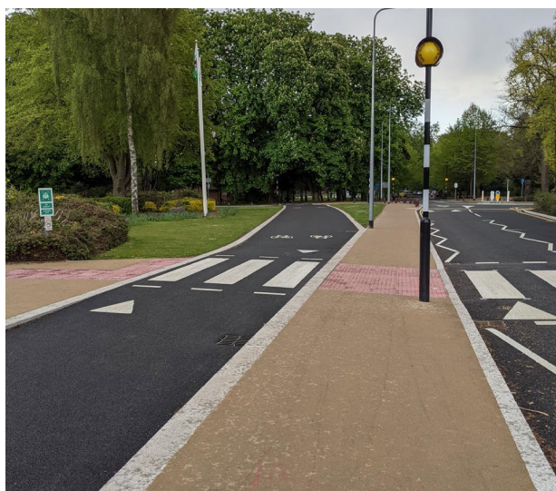
Figure 12.8 – Zebra crossing of cycle track, Cardiff
