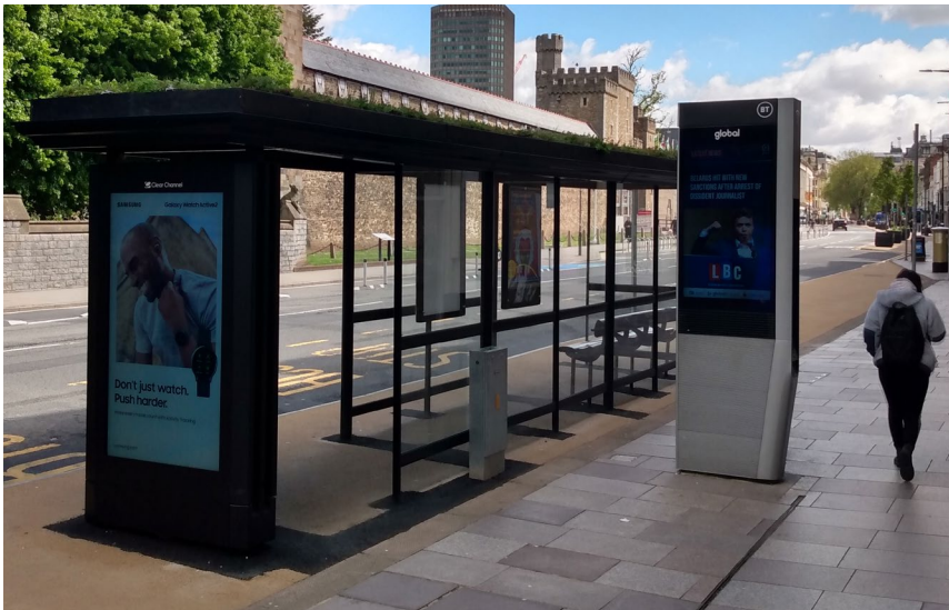
Figure 13.1 – Green roof on bus stop
