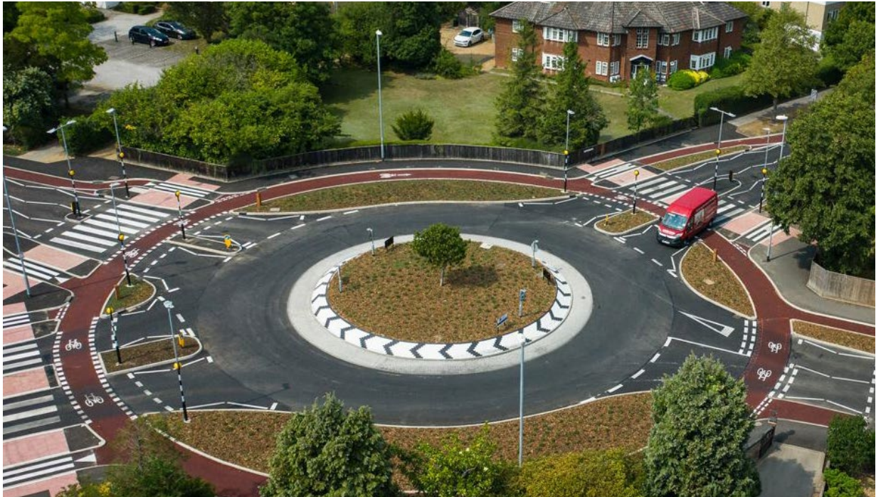
Figure 12.25 – Dutch style roundabout in Cambridge
