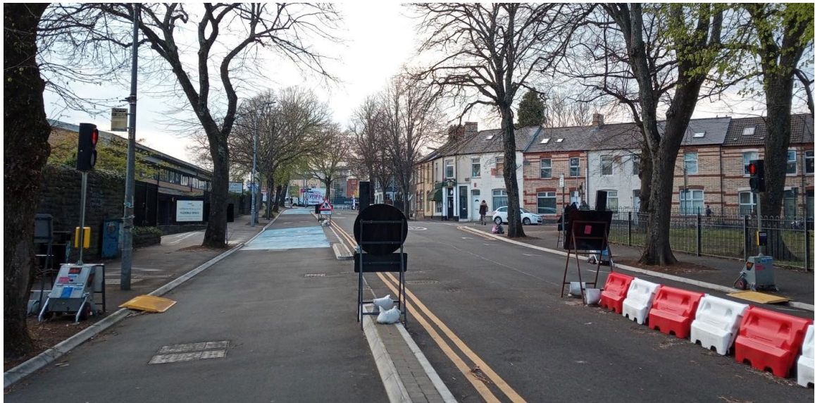
Figure 15.13 – Streetworks with active travel provision
