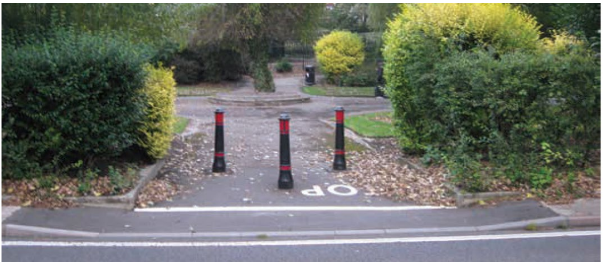
Figure 15.2 – Access control using bollards
