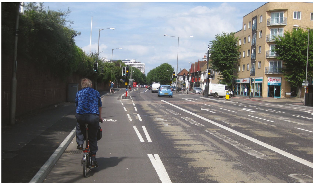
Figure 12.14 – Ahead-only cycle bypass
