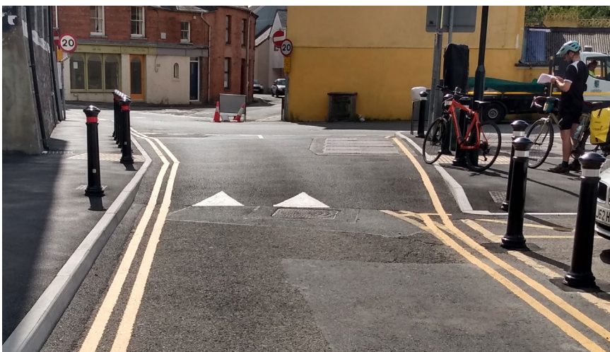
Figure 11.3 – Example of a raised table with tactile crossing point in Cardigan, Ceredigion
