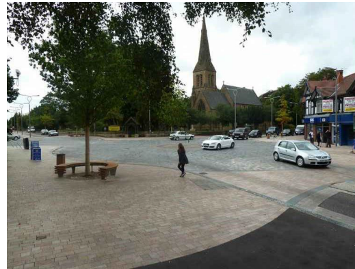
Poynton, Cheshire Double Junction, each designed to encourage circulatory priority, with courtesy crossings, carrying circa 26,000 vehicles per day overall
