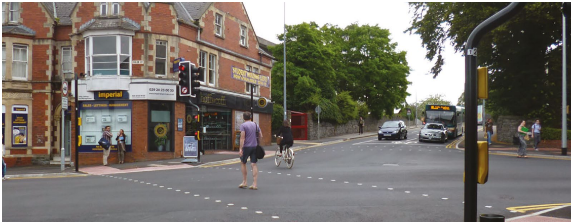
Figure 12.13 – Signalised diagonal pedestrian and cycle crossing, Cardiff
