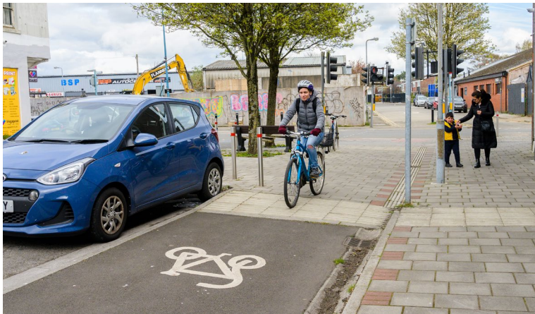
Figure 11.15 – Stepped cycle track, Cardiff
