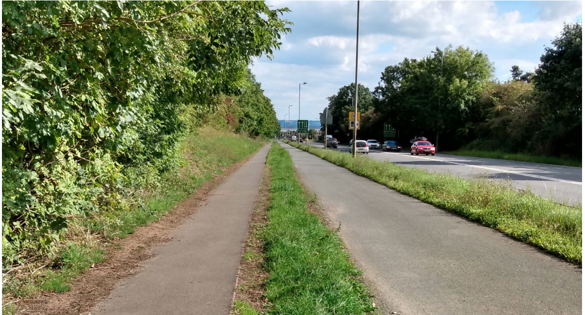
Figure 11.11 - Cycle track and pedestrian footway alongside road, separated by grass verge
