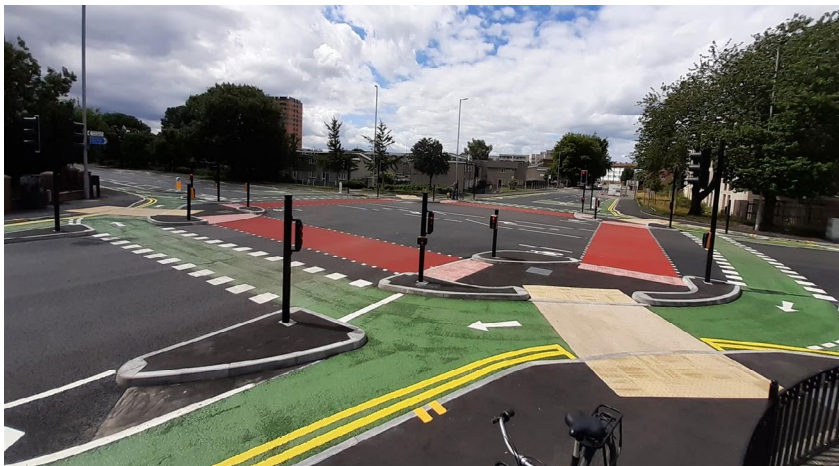
Figure 12.19 – Four way signal controlled junction with pedestrian and cycle provision. Commonly referred to as a cyclops junction.
