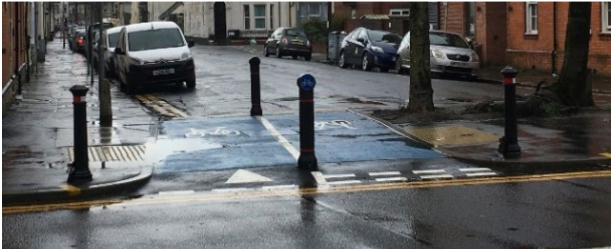
Figure 11.4 – Modal filter allowing pedestrian and cyclist access through an area restricted to motor vehicles
