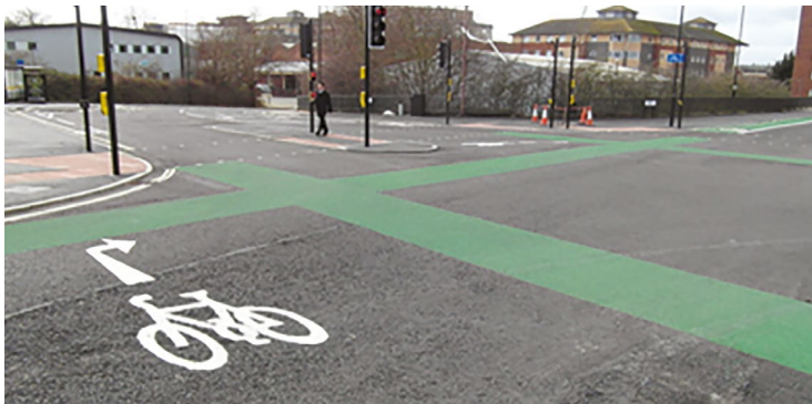
Figure 12.18 – Two stage right turn signalised junction
