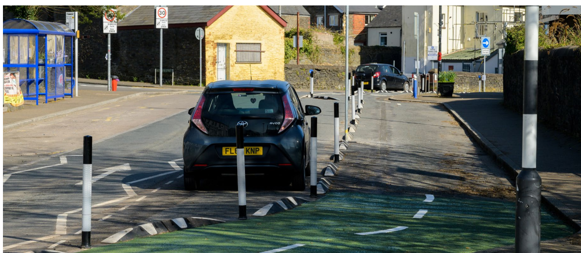
Figure 11.14 – Two-way cycle lane using light separation
