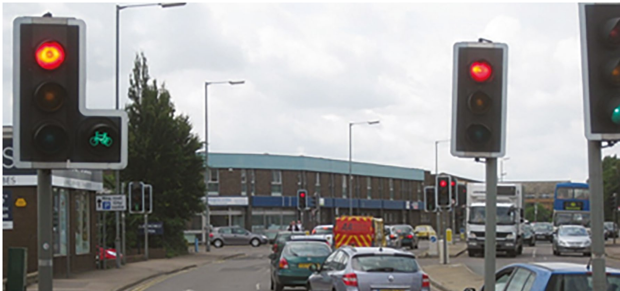
Figure 12.12 – Permanent green signal at bus gate
