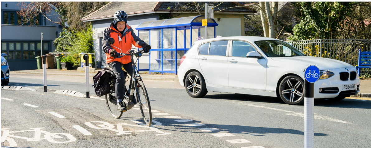
Figure 11.9 – Reallocation of road space using light separation features, Ystrad Mynach
