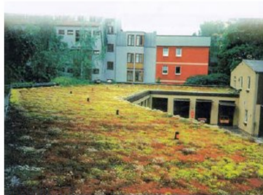
Sedum roof on garages, Germany
