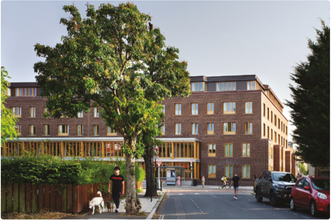
Appleby Blue—elevation to the high street, with adjacent bus stop
