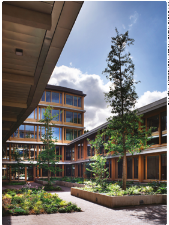
Wetherford Watson Mann Architects/Phillip Vile
